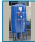
Pressure Filters Tank
