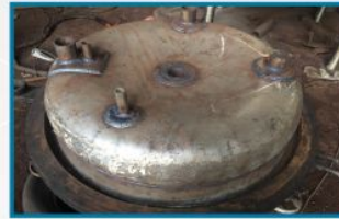
Gas Carburising Furnace
